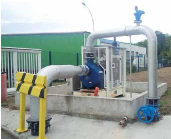
Motor-driven pump for the pumping of leachate 400 m3h
