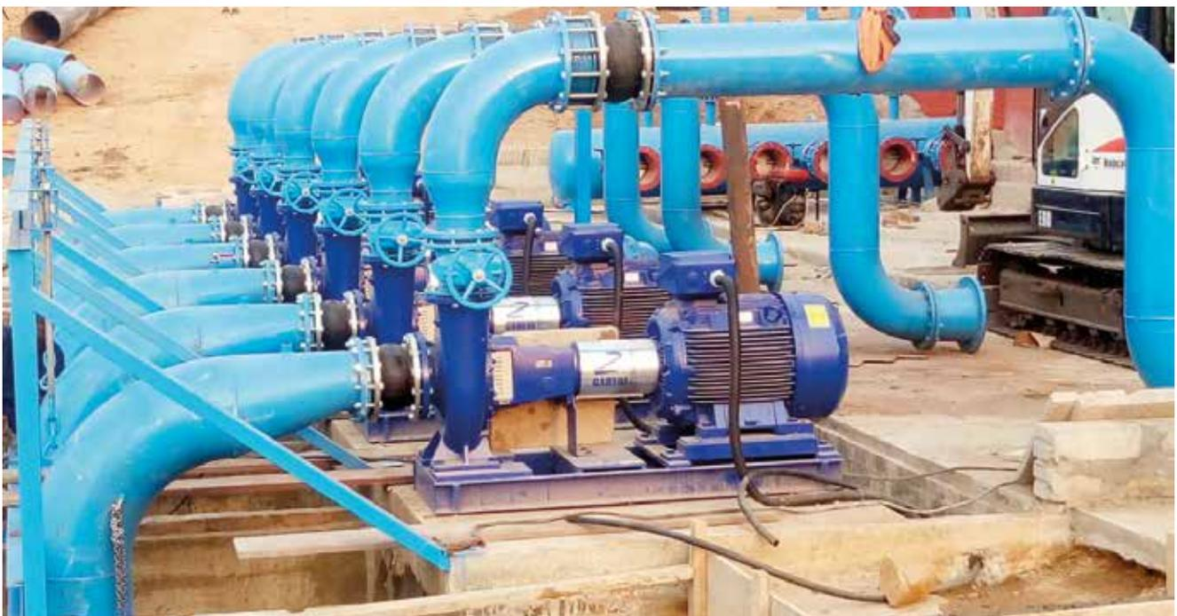
Pumping station with electric pumps being installed
